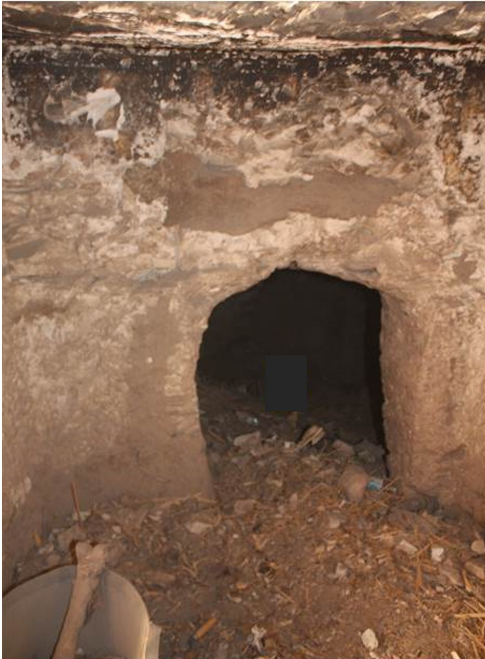
Fig.19 The opening with gabled roof between TT362 and TT363.
