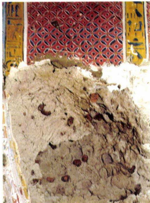
6. Detail from the north-western corner of the ceiling of the transverse-hall. Donkey excrements and their imprints and traces of the handwork can be seen in the mortar.
