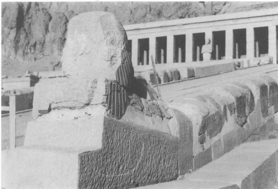
3. Left-hand balustrade of the ramp leading to the upper terrace of the temple of Hatshepsut at Deir el-Bahri (photograph by I. Shaw)
